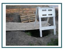
This photo is an example of how **NOT** to set-up a barrier at an excavation.
